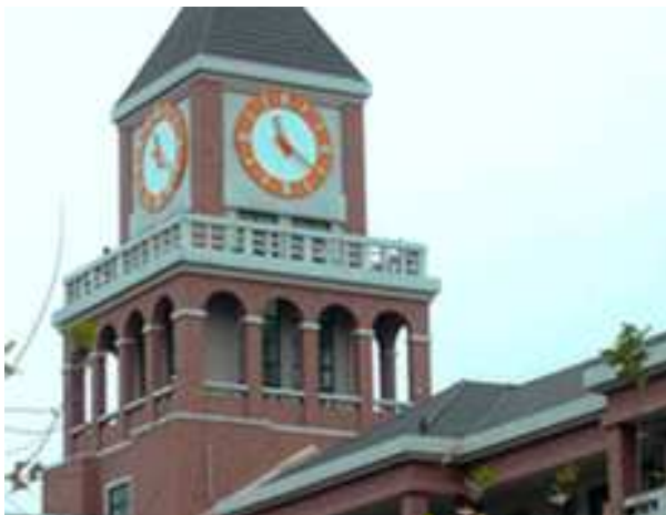
Shanghai Fu Shan foreign language university φ2.5m 4faces Tower Clock LED Lighting
